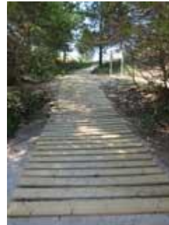
Sample Boardwalk - Photo courtesy of Pinery Prov. Park
